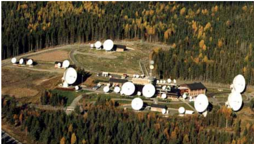
Nittedal Earth Station, Norway
